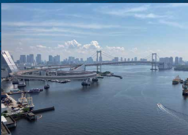
The distinctive loop design on the Shibaura side of the Rainbow Bridge (toward the city center)
